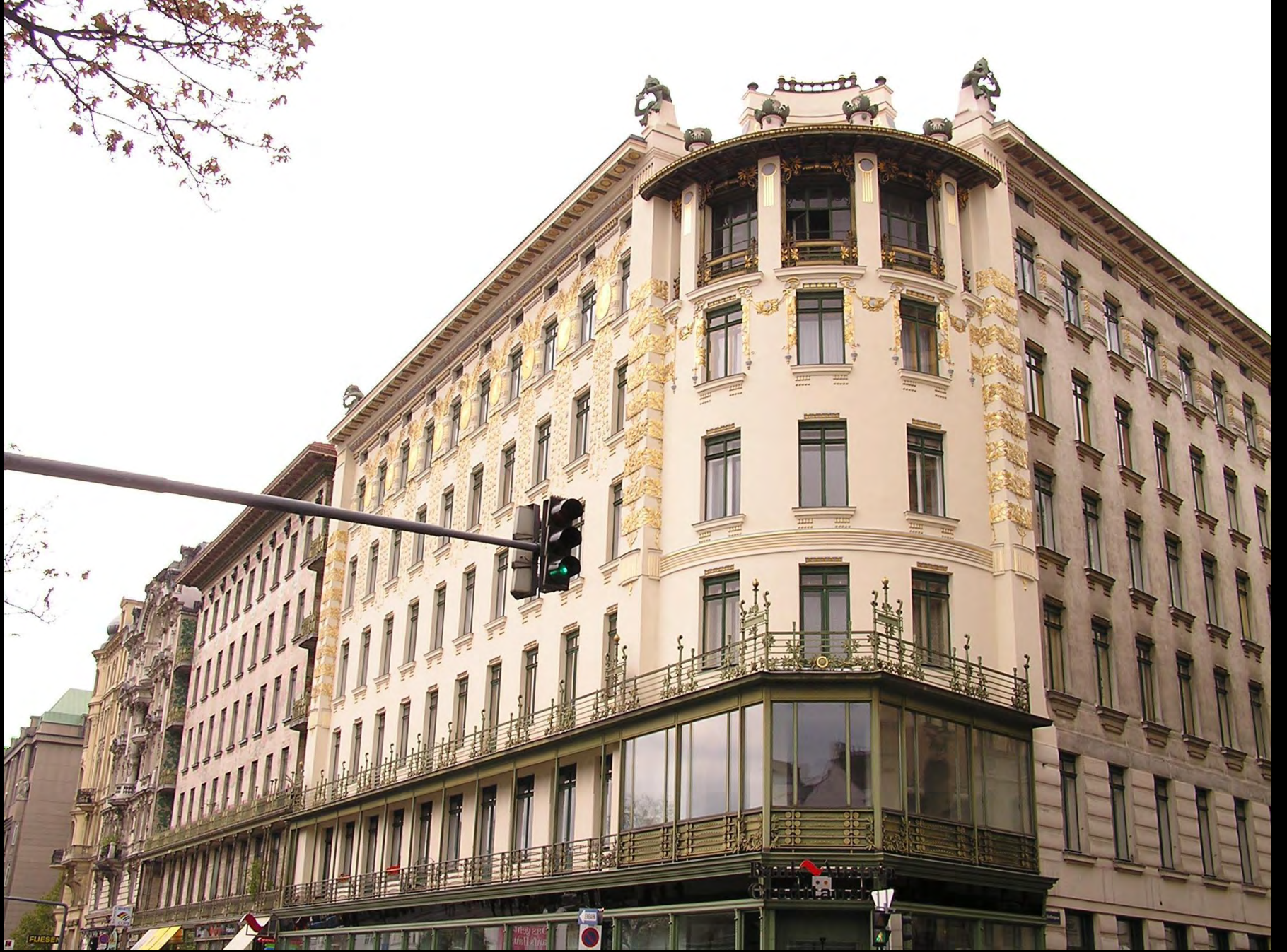
Otto Wagner, Apartment Houses, Linke Wienzeile 38 (front) - 40 (back), 1898-9
