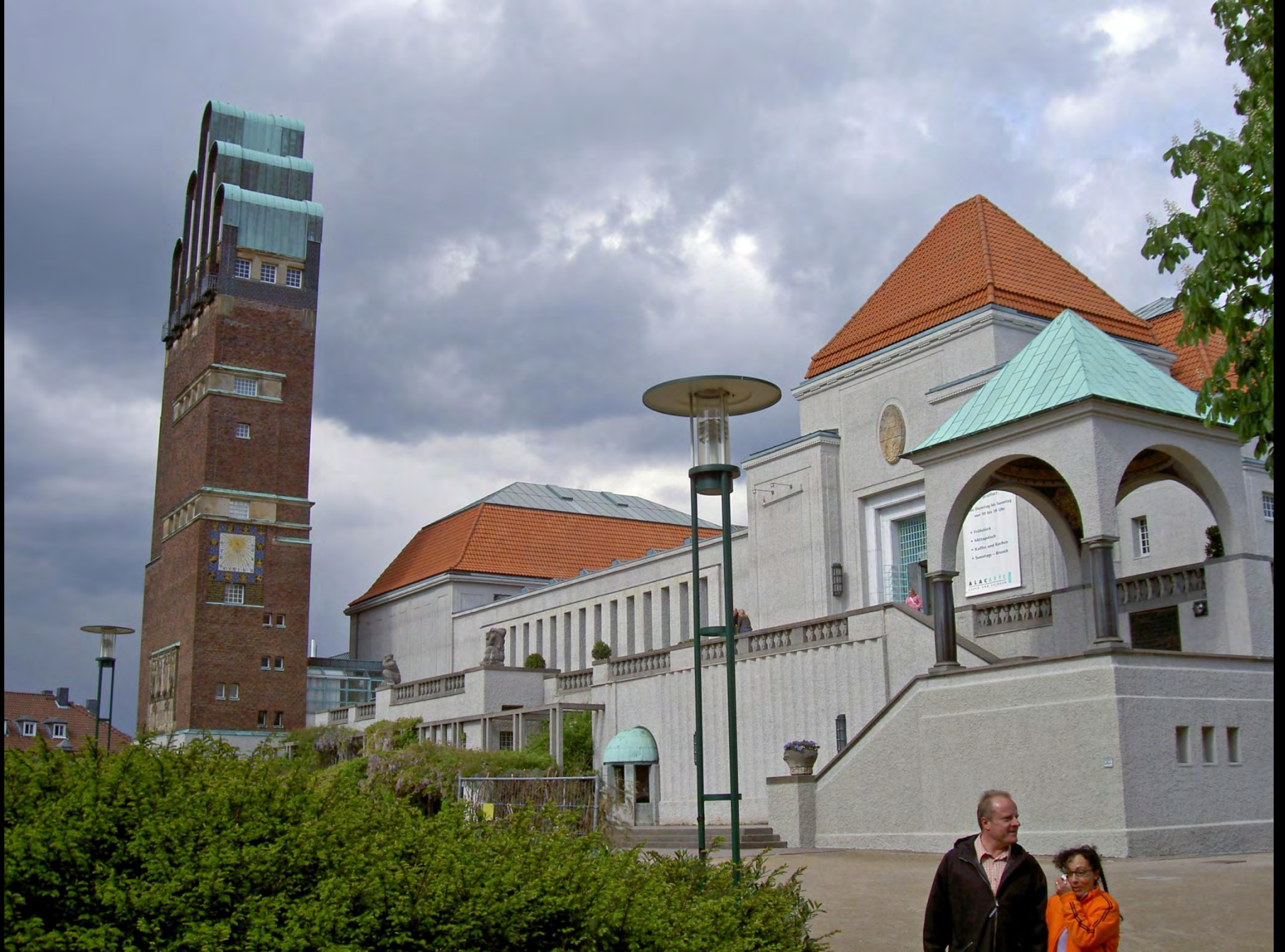
Joseph Maria Olbrich, Mathildenhöhe, Wedding Tower and Exhibition Building, Darmstadt , Germany, 1905-08. c
